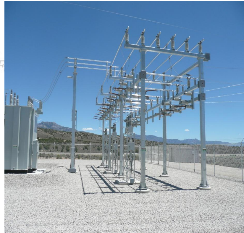
New Pescio sub 34.5 kv serving Railroad Valley & Duckwater
